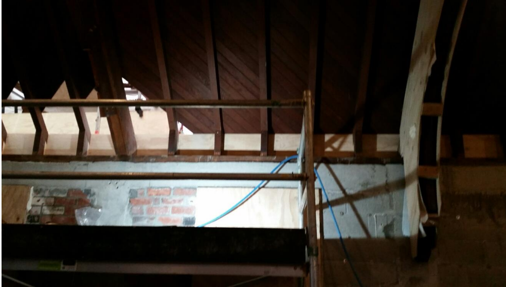
The original timber sarking to the roof has now been re-instated.
