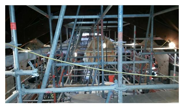
View of the Chapel Nave looking back towards the front entrance to the building. The scaffold propping has supported the roof independent of the building whilst the strengthening works have been completed. The propping will be removed the first week of May now that the building and roof are re-connected.
