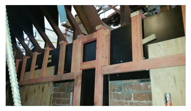
The black panels indicate the boxing to the vertical buttress columns and the horizontal ring beams at the time of the concrete pour to the nave areas. All reinforced concrete to the Nave has been completed.
