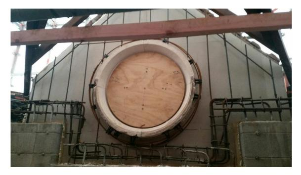
View of new reinforcing being installed to the round stained-glass window in the Chancel.
