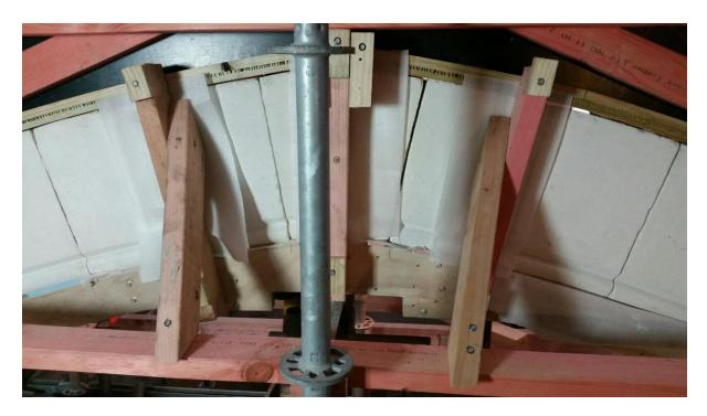
The reinstallation of the Oamaru Limestone Arch to the Chancel has now started. The existing stone was carefully deconstructed and has now been installed back to its original position.
